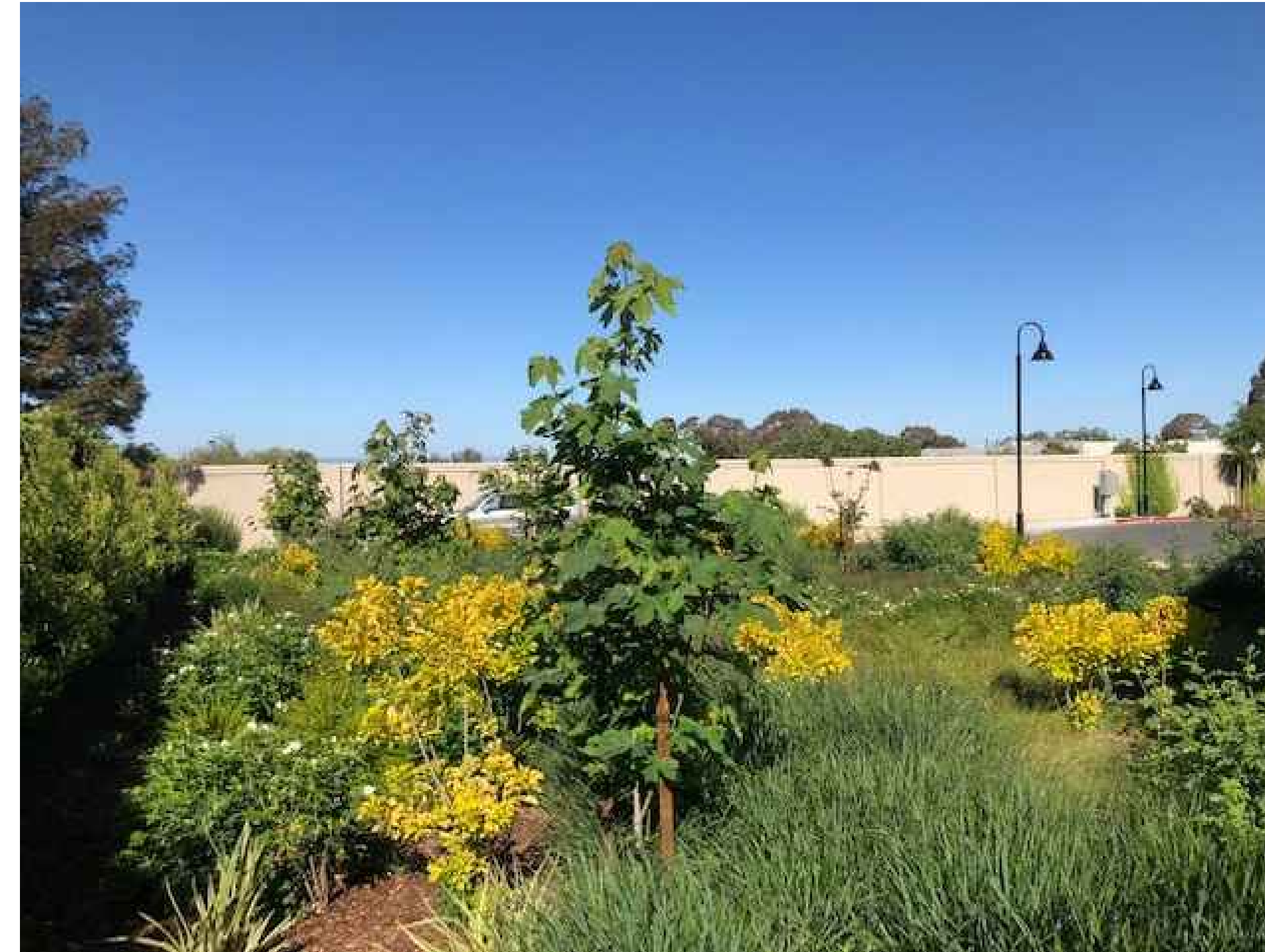
PLANTING IN BIO RETENTION AREAS - A MIX OF GRASSES, SHRUBS AND TREES PER THE STORMWATER C3 GUIDEBOOK PLANT LISTS
